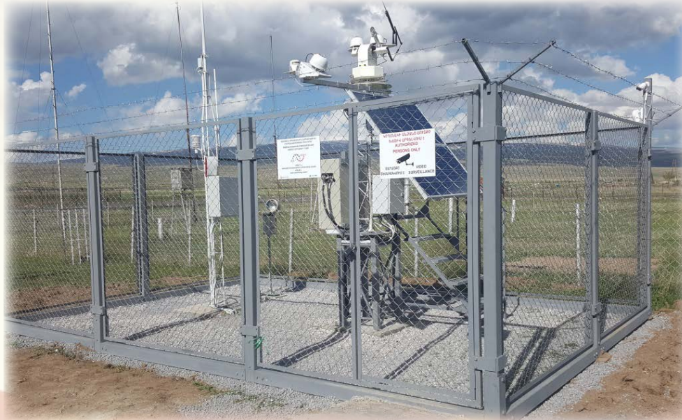
Typical field installation of the SEMS-3000 System with solar sensors mounted on the sun tracker, plus meteorological mast, datalogger and power supply for autonomous unattended operation of the whole system
